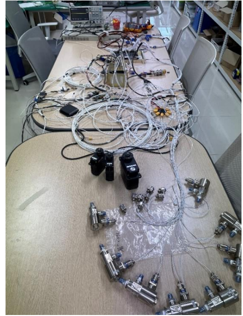
Fig. 6. Valve System Control Test
